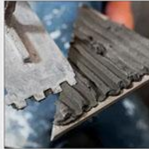
Cement Laying on Tile
