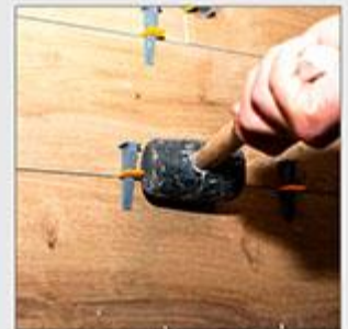
Remove Wedges Ones It Dry
