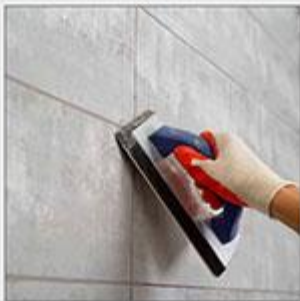
Joint Grouting
