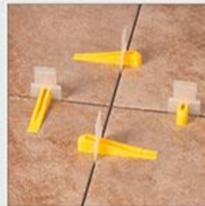
After Lavelling Process leave Int For 8-10 Hrs
