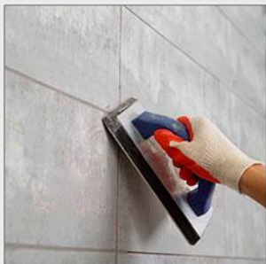
Joint Grouting
