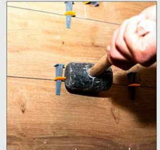
Remove Wedges Ones It Dry
