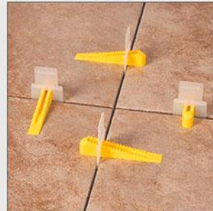
After Lavelling Process leave Int For 8-10 Hrs
