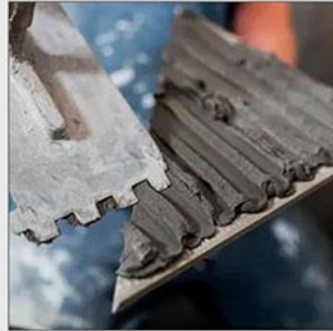
Cement Laying on Tile
